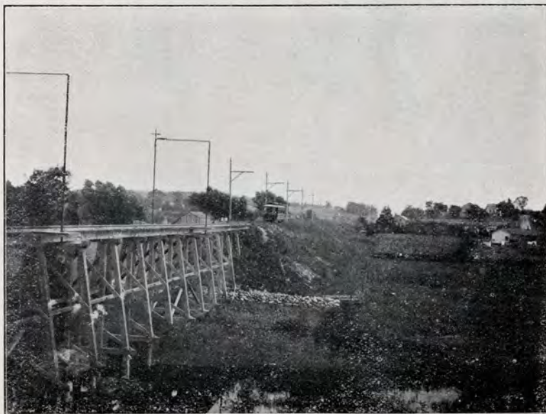
TRESTLE ON ROAD TO WAVERLY PARK.
