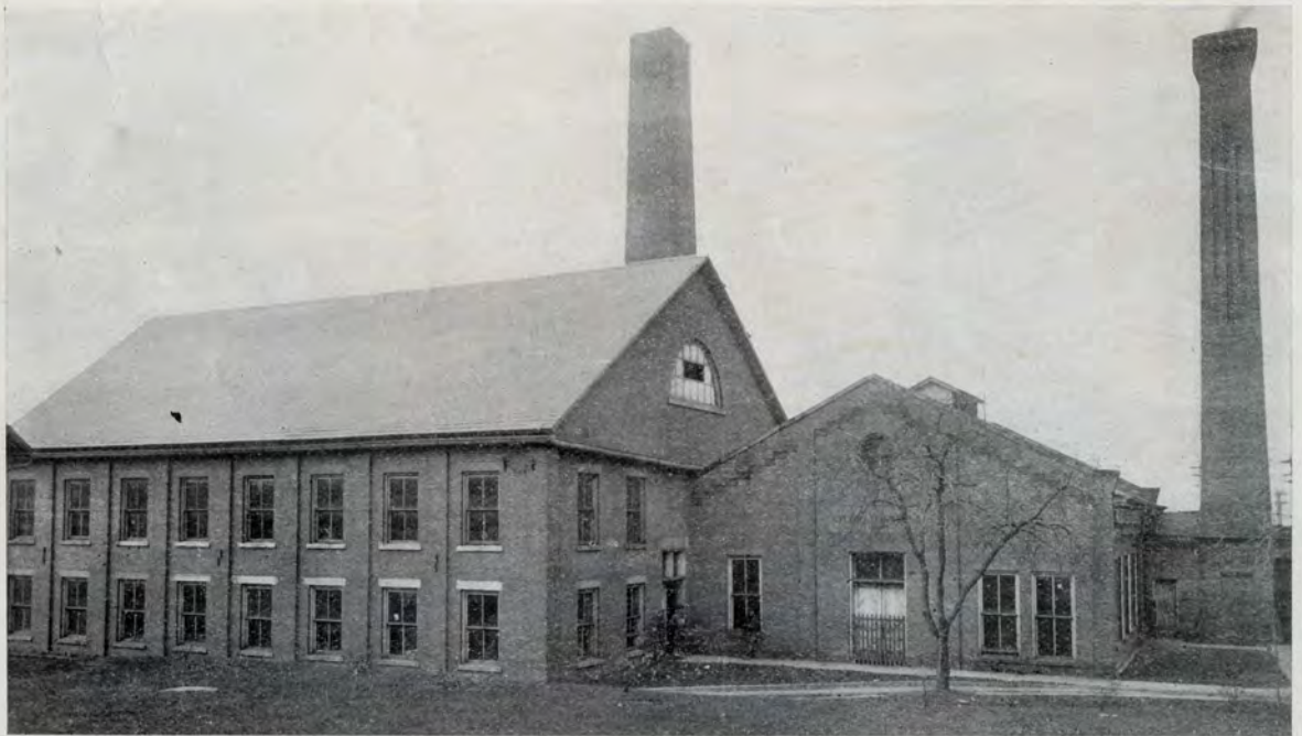
MUNICIPAL LIGHT AND WATER PLANT.
