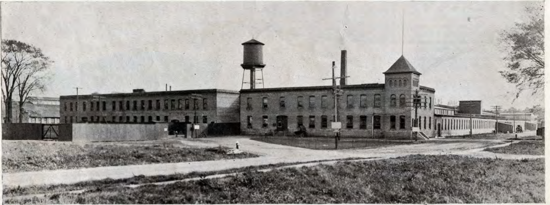
OLDS MOTOR WORKS.
